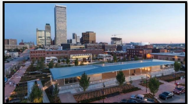
Guthrie Green pavilion having 192 solar panels installed by Harvest Solar Energy providing power for park concessions, lights and stage.
